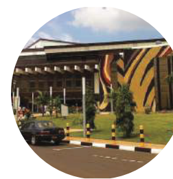
5 Kigali City Airport 23 min (10 km)
